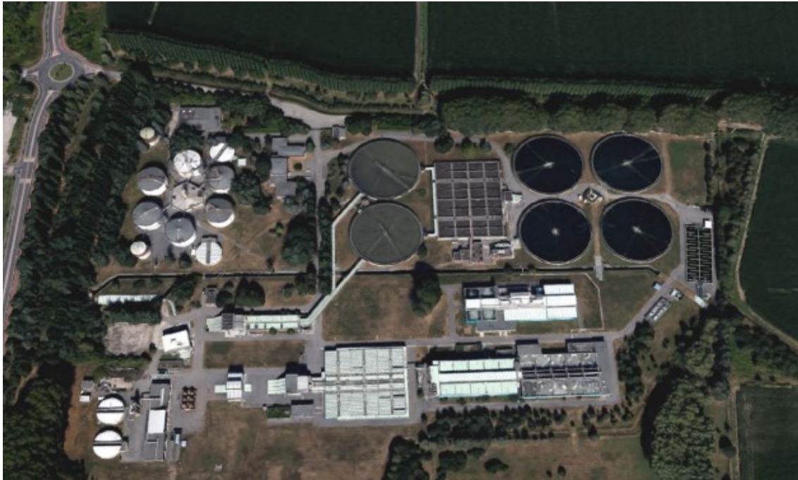
Figure 3-1. Aerial view of Peschiera Borromeo WWTP
