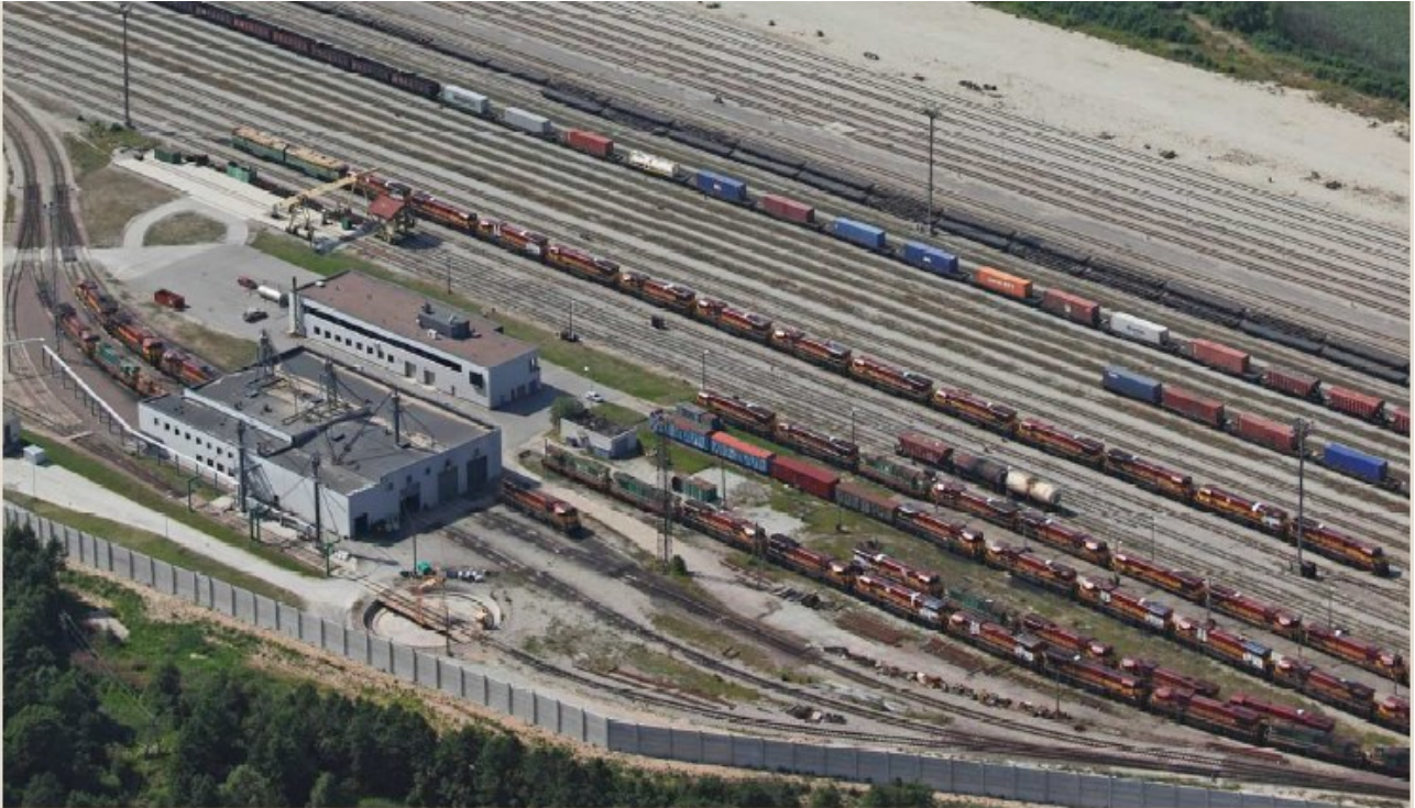
Figure 8: Noise barrier at Tallinn port (ESPO, 2013)
