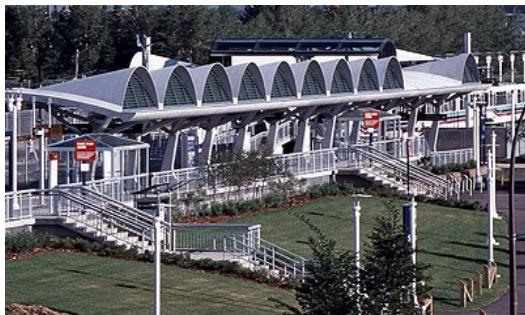
Fig. 5 – RLT station, Shawnessy, Canada
