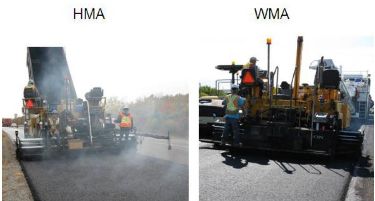
Figure 14. Visible asphalt fumes at the asphalt paver (HMA vs WMA) [34].
