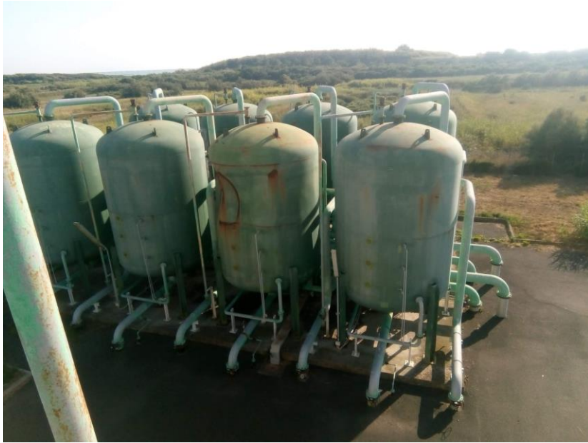
Figure 3: Unit of active carbons filtrations in the current Aretusa plant
