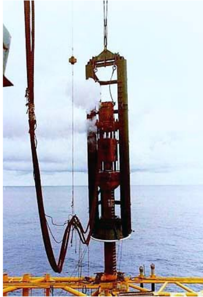
Figure 8 Steam hammer
