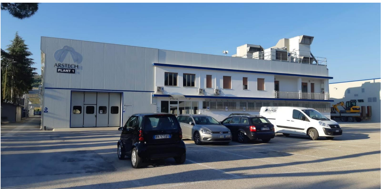
(fig. 1.1 stabilimento ArsTech a Colonnella, plant 1)
