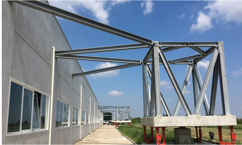
Figura 3.16: Capannone "TexPoint" – Gonzaga (MN)
