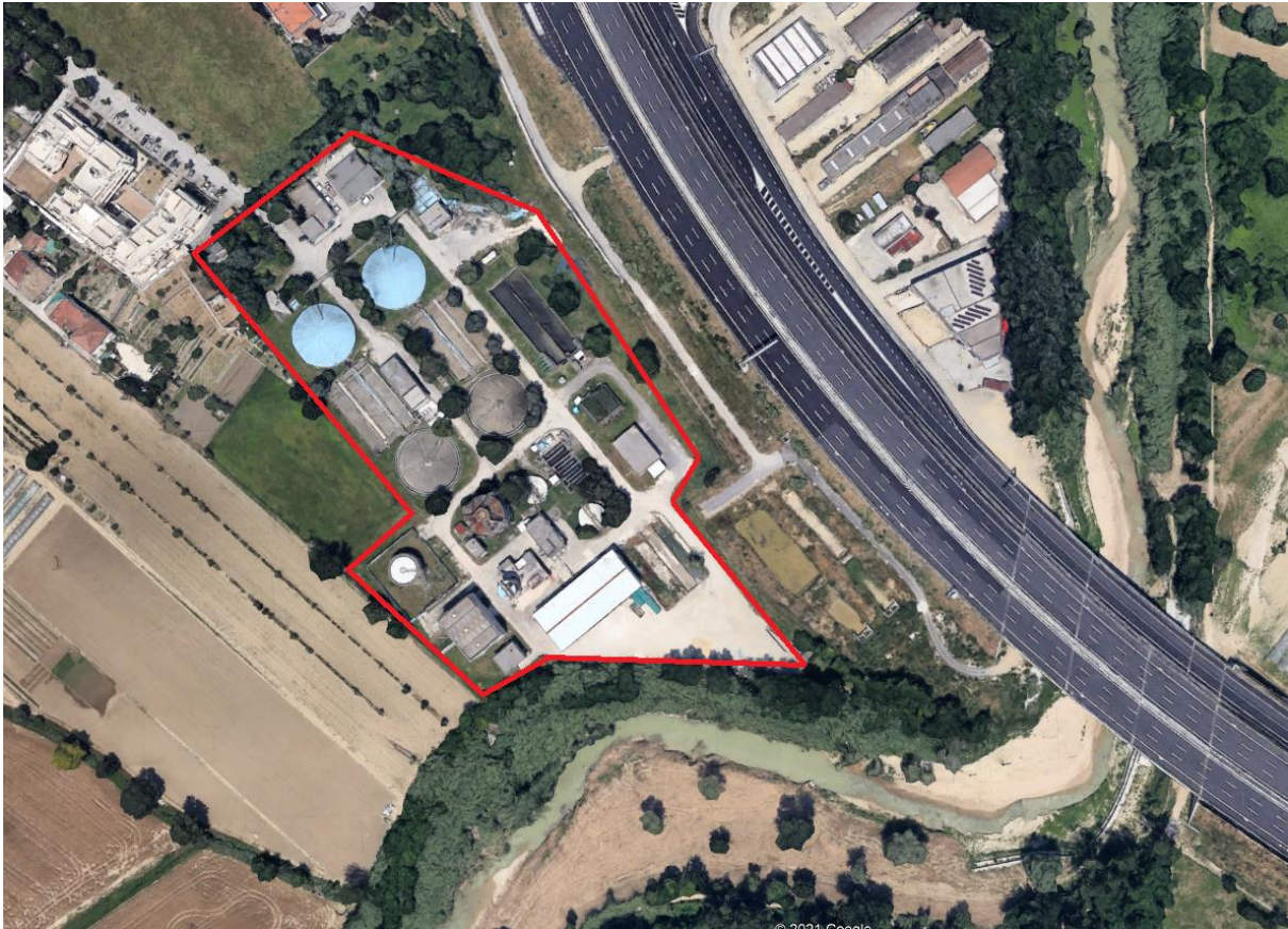
Figure 56. Senigallia wastewater treatment plant top view.
