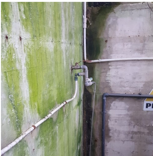
Figure 33 Ozonation effluent sampling point (1)
