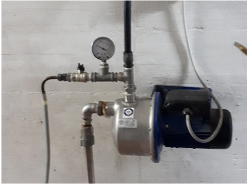
Figure 31 Sand filters effluent sampling point (1)
