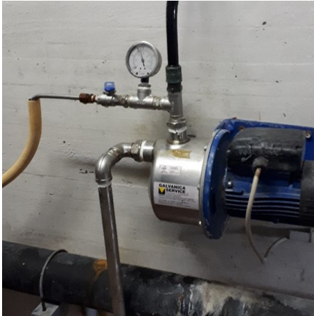
Figure 35 Activated carbon effluent sampling point (1)
