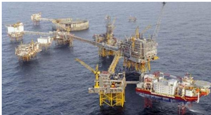
Figura 1.1: Piattaforma offshore "Shallow Water Complex"
