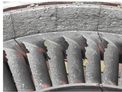
(b) Foreign object damage (FOD) on a gas turbine
