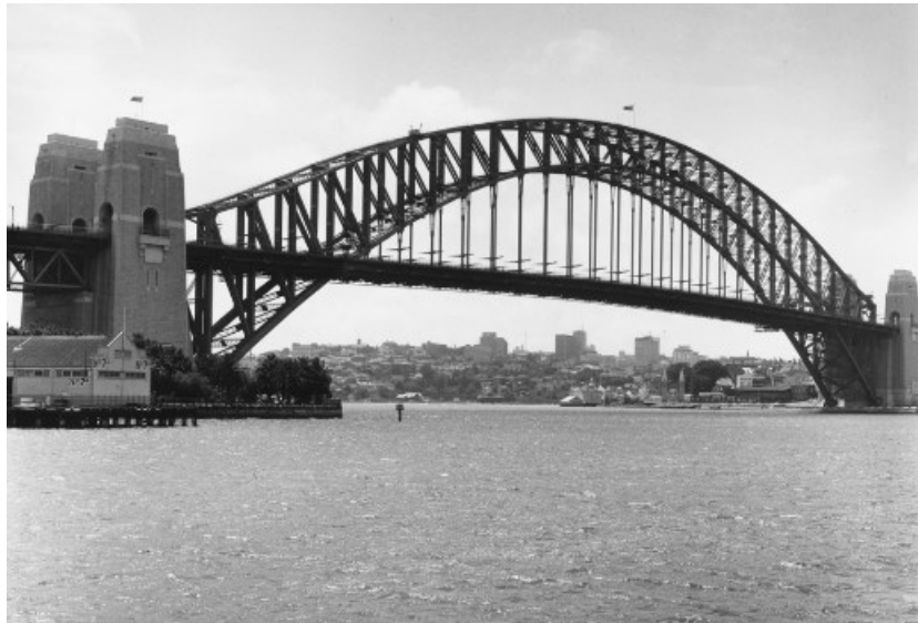
Figura 3- Sydney Harbour Bridge 1932.
