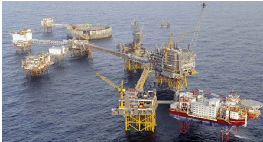
Figura 3.4: Piattaforma offshore “Shallow Water Complex”.
