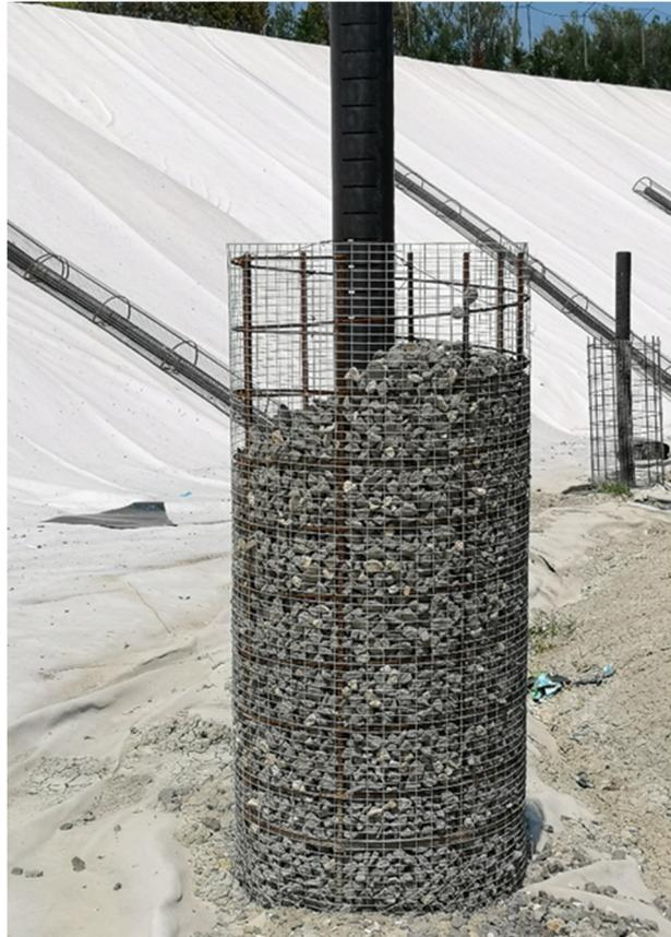
*FIGURA 5 - POZZO VERTICALE CON COLONNA DI INERTI E RETE METALLICA DI CONTENIMENTO – FONTE: “SMARTENVI PROJECT - SMART DECISION TOOLS FOR REDUCING HAZARDS TO OUR ENVIRONMENT AND WATER RESOURCES BY REHABILITATING OPEN DUMPS” – ASET SPA*
