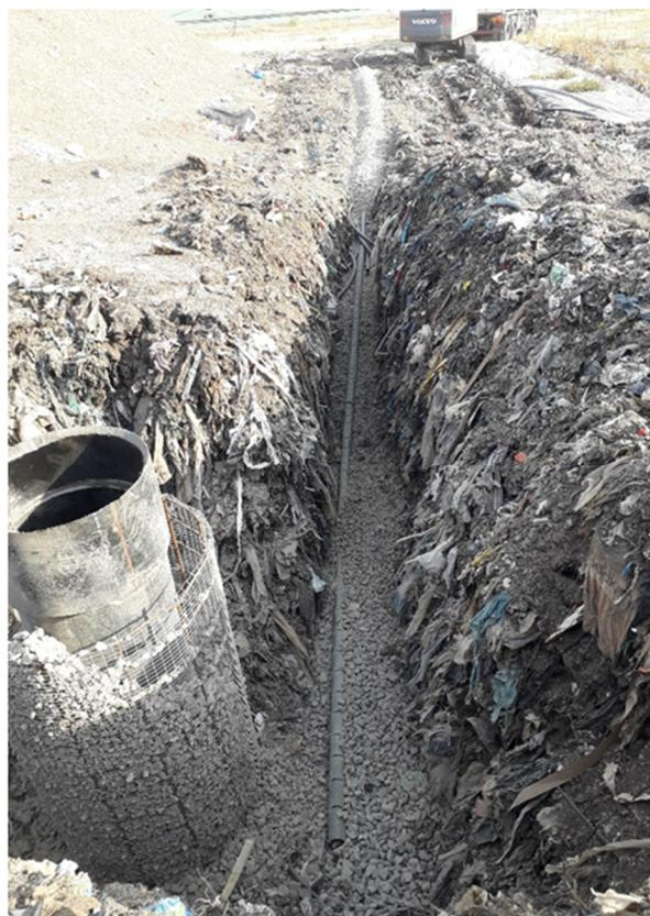
*FIGURA 6 - DRENAGGI SUB-ORIZZONTALI – FONTE: “SMARTENVI PROJECT - SMART DECISION TOOLS FOR REDUCING HAZARDS TO OUR ENVIRONMENT AND WATER RESOURCES BY REHABILITATING OPEN DUMPS” – ASET SPA*
