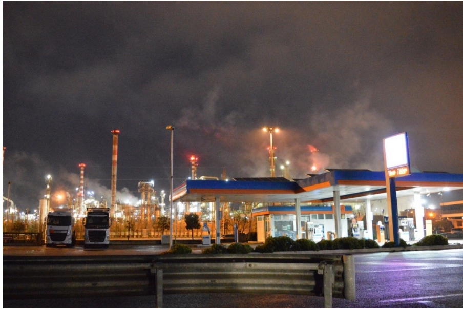
Figure 8. Plume emitted by API refinery in Falconara Marittima, Italy, aloft due to PBL stratification, lightly rising due to residual ground heat flux (Cronache Ancona, 2024.)
