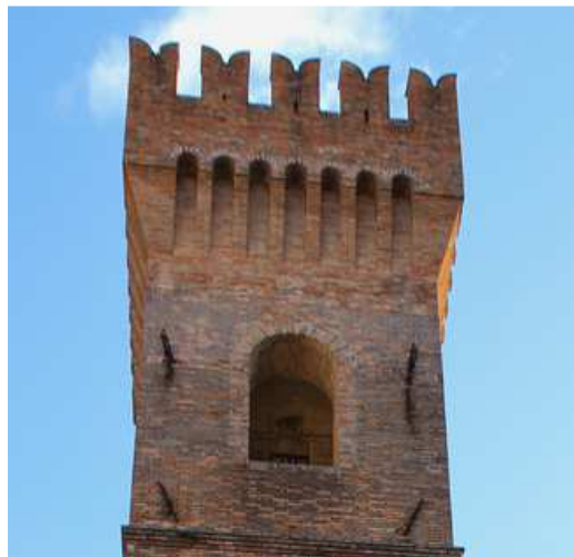
Figure 4-15 – A photo of the belfry of the Civic Tower
