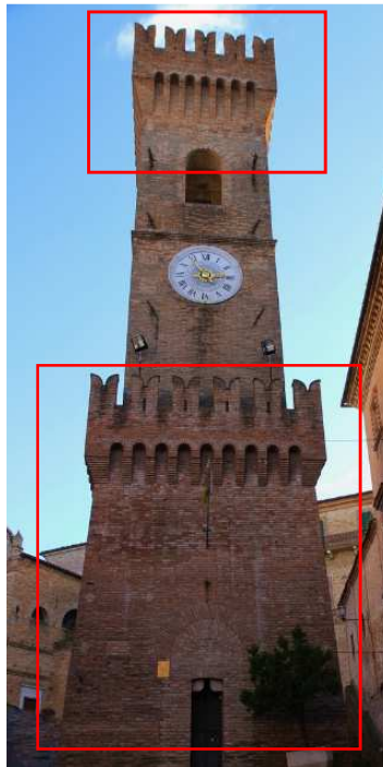
Figure 4-9 – A photo of the main facade of the Civic Tower. The basement and the top of the tower, highlighted by red rectangles, were probably reconstructed in the fifties’: this is visible from the different tonality of colour of these masonry parts.
