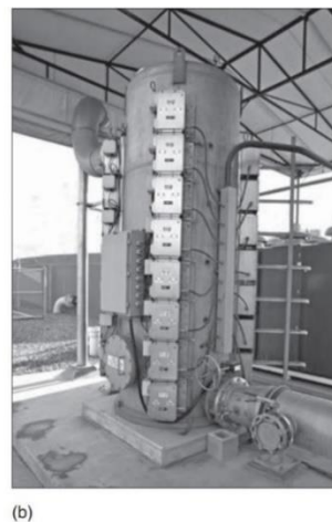
Hydrogen peroxide and UV radiation advanced oxidation process (a) schematic diagram (from Crittenden et al., 2012) and (b) photograph of typical vertical flow UV reactor.
