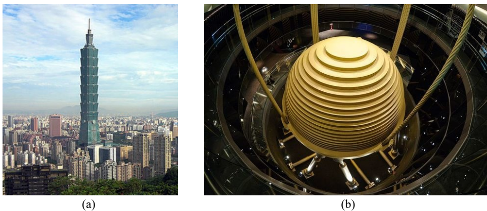
Figure 4. 2: (a) The building Tapei 101 (Taiwan). (b) The tuned mass damper inside the building Tapei 101.
