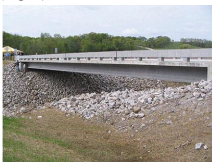
Fig. 3 - Wapello County Bridge (Iowa, USA)
