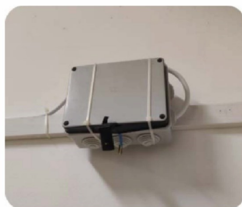
Figura 27_ Sensore people counter installato a Falconara
