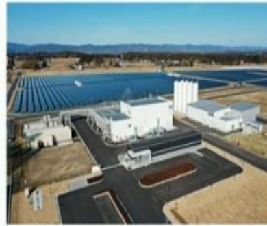
Largest electrolyzer in the world (10 MW) powered by a by a photovoltaic plant (20 MW, 18 hectares)
