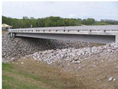
Figura 3 - Wapello County Bridge (Iowa, USA)
