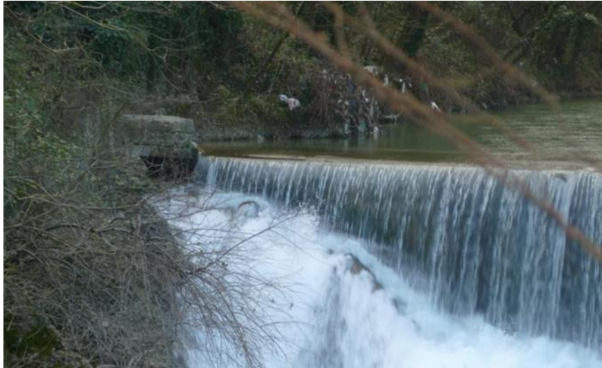
FIGURE 36: LATERAL VIEW OF THE OLD INTAKE STRUCTURE
