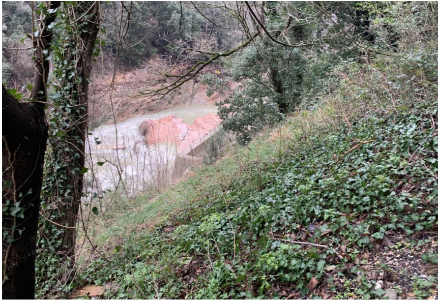
FIGURE 47: TRAIL FOR THE ACCESS POINT TO THE PLANT
