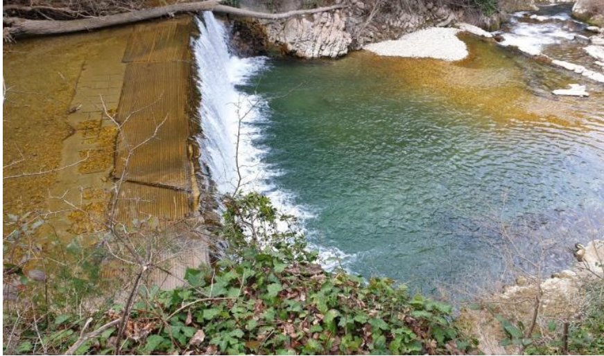
FIGURE 15: FIRST REGULAR UPSTREAM WEIR
