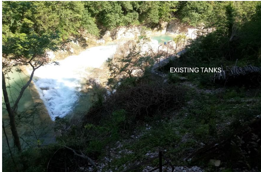
FIGURE 18: VIEW FROM THE TOP OF THE EXISTING TANKS
