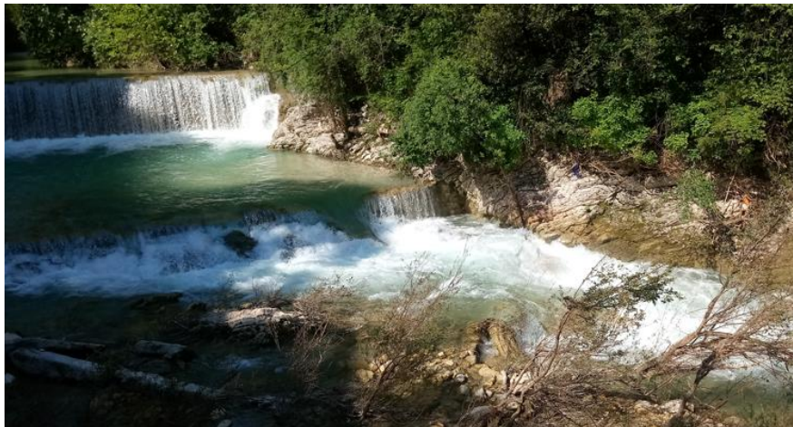
FIGURE 16: SECOND IRREGULAR DOWNSTREAM WEIR
