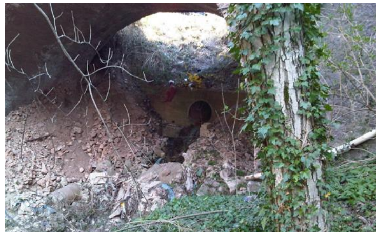
FIGURE 44: VIEW OF THE EXISTING DISCHARGE
