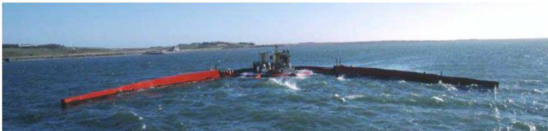
*Fig.1.8 Wave Dragon prototype (Overtopping Wave Energy Converters: general aspects and stage of development. (2011). Giovanna Bevilacqua Barbara Zanuttigh. [http://amsacta.unibo.it/3062/1/overtopping\\_devicex.pdf](http://amsacta.unibo.it/3062/1/overtopping_devicex.pdf))*
