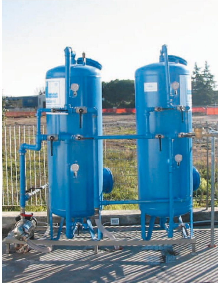
Figure 49: example of two column filtration system (Boer group)
