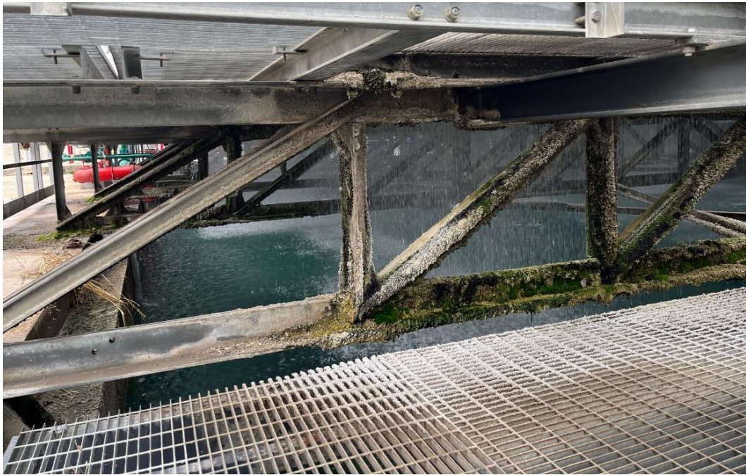
Figure 44: focus water cooling through the spray nozzles
