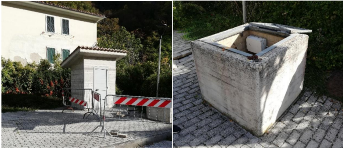
Figure 4. a) Instability phenomena in correspondence of the pumping well; b) pumping well (modified from Lenci, 2021).
