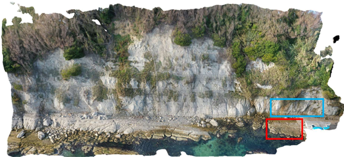
Figure 27 - Sampling windows: horizontal (red) and vertical (blue) portion of the cliff.
