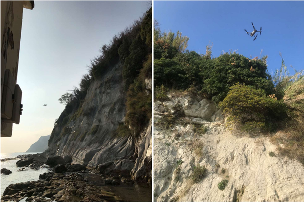
Figure 18 - Mavic 2 Pro drone flights: acquisition of the cliff surface.
