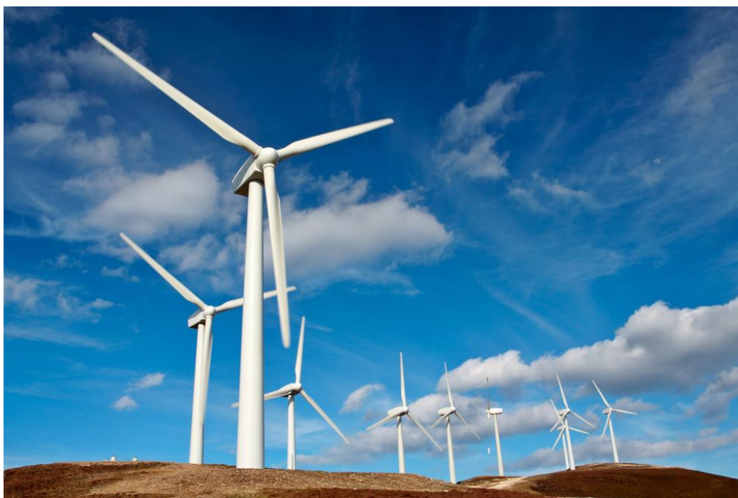
Fig.3 – Wind turbines farm [3]
