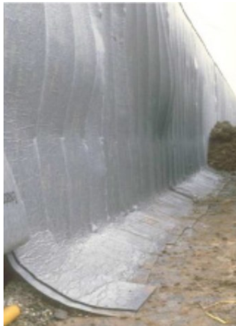
Fig. 29 Posa in opera verticale
