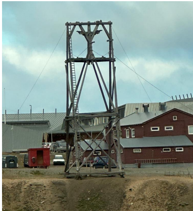
Figure 1.2 Medium cableway post reference structure
