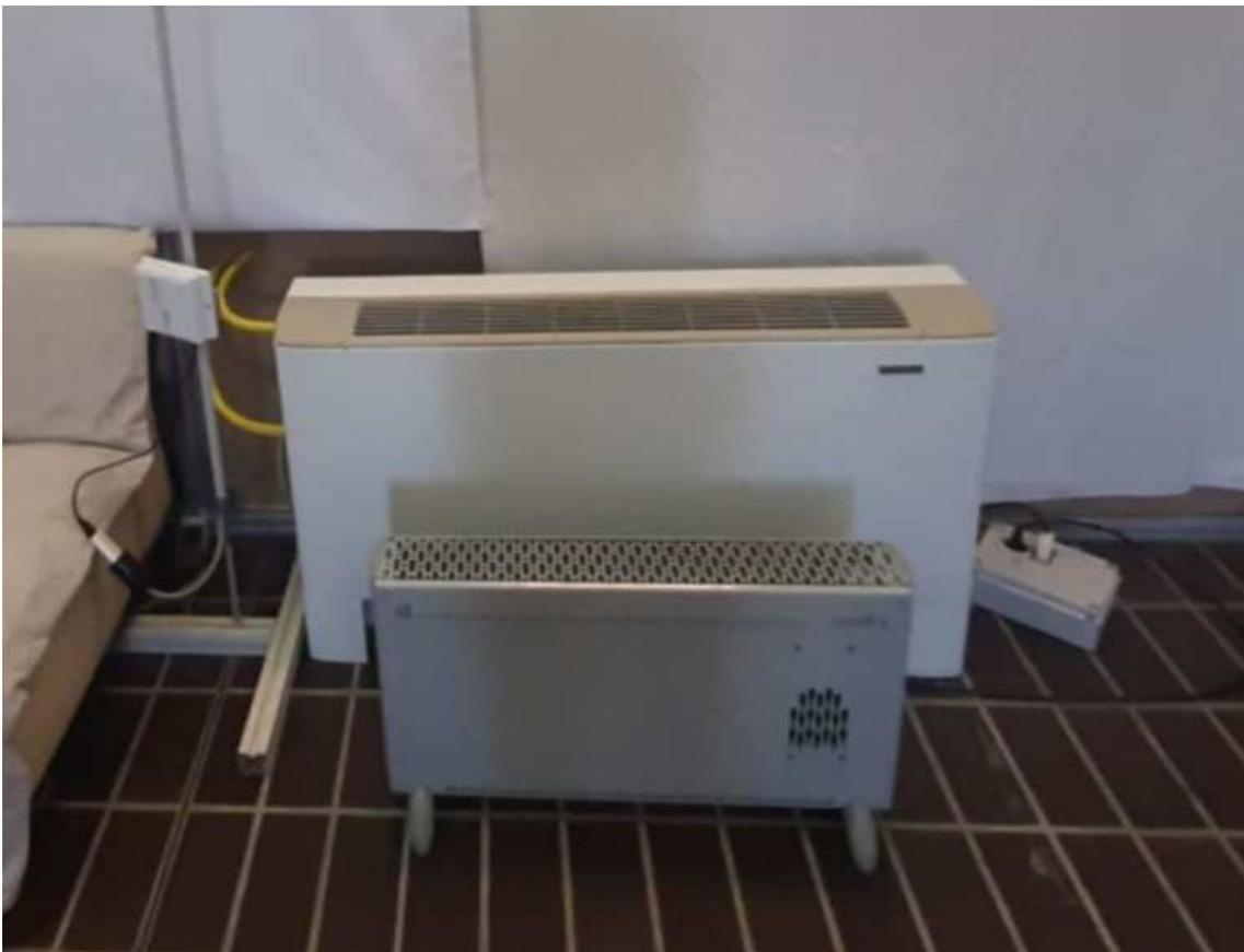
**Figura 6.** Fan-coil e stufa
